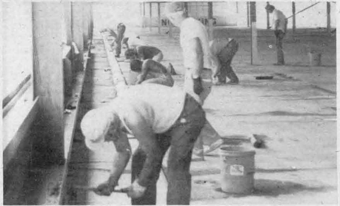
ARTHRTIC PARKING LOT: Strengthening the joints of Parking Lot four is one preparation being made for fall students. The lot will be closed for about one month. [Photo by Douglas Dieckman]
